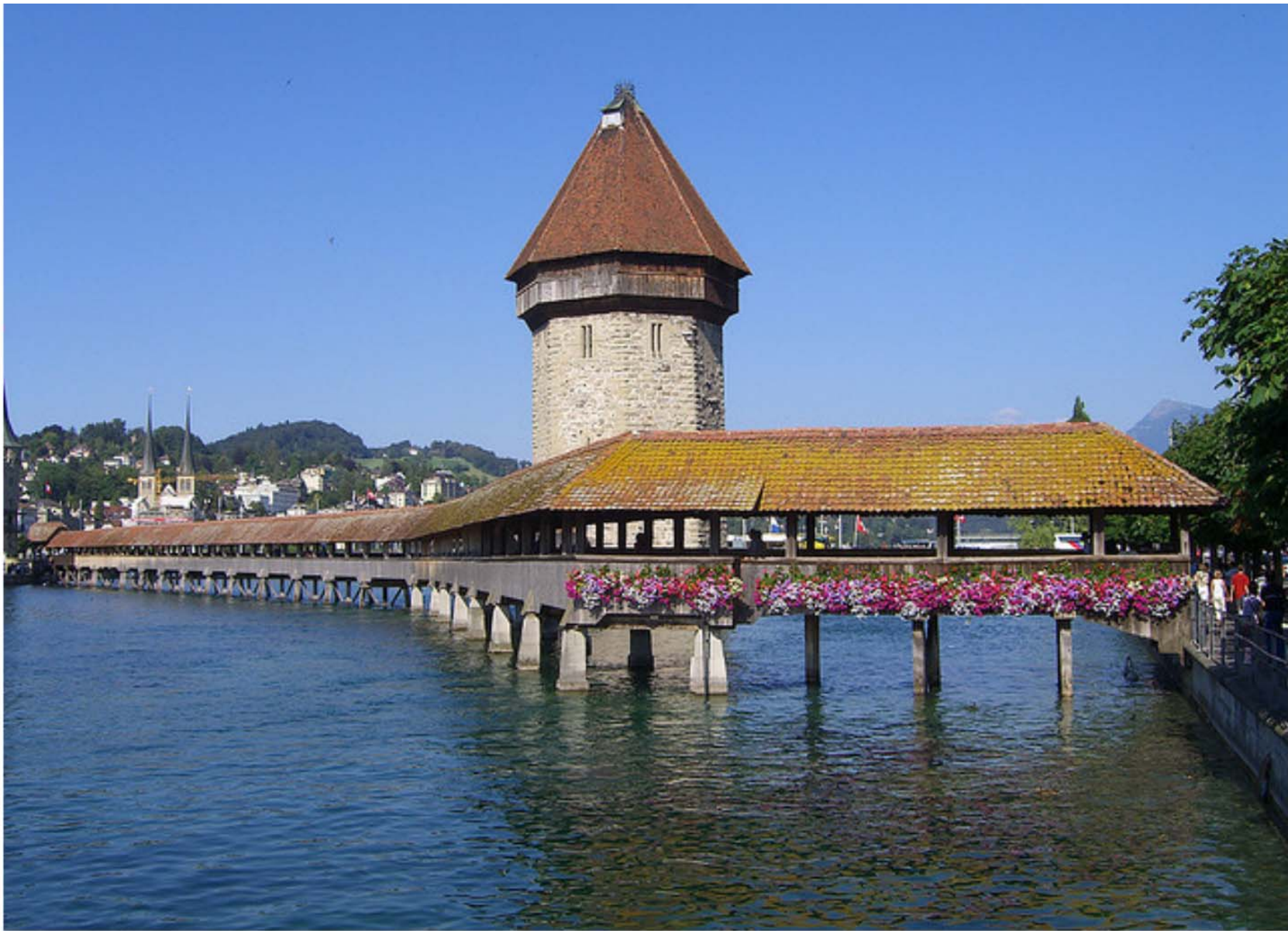
Chapel Bridge, Switzerland
