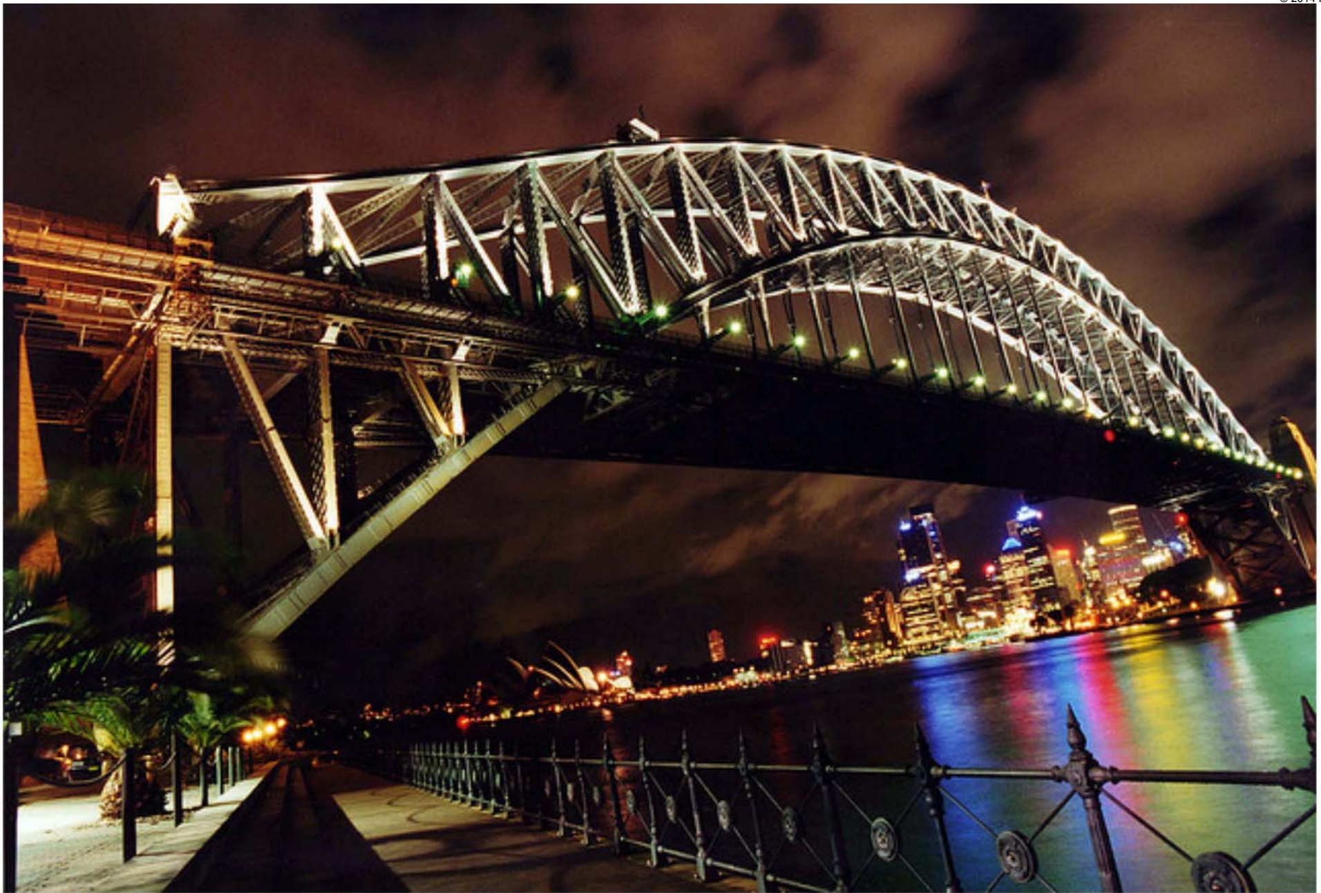
Sydney Harbour Bridge
