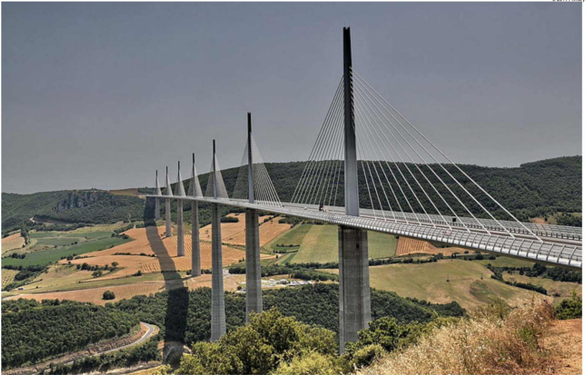
Milau Bridge, France
